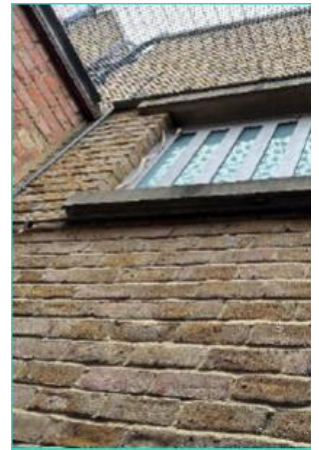
Holding cell windows
